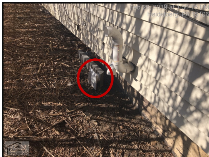
Figure 12 The dryer exhaust vent is discharging at ground level.
