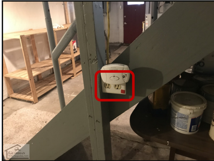
Figure 35 One three-prong electrical outlet, along the basement stairway, has reversed polarity (i.e. the hot and neutral wires are wired backwards).
