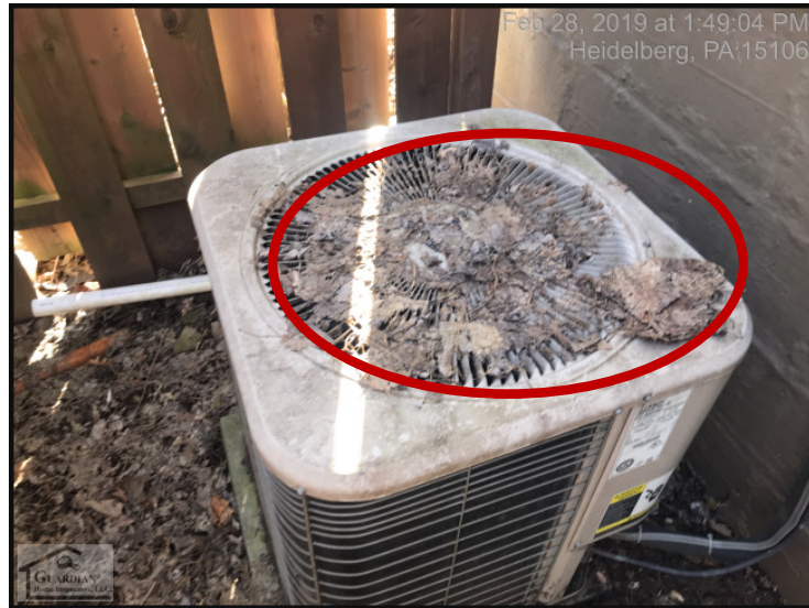
Figure 9 The condensing coil fins, on the exterior AC unit, are significantly dirty.
