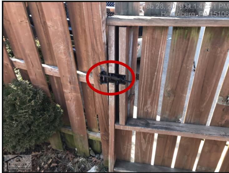
Figure 1 The gate and latch hardware on the fence is in poor operating condition.
