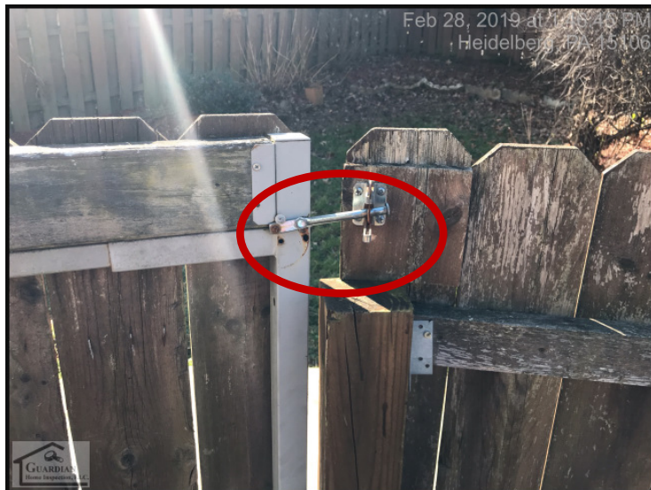
Figure 2 The gate and latch hardware on the fence is in poor operating condition.
