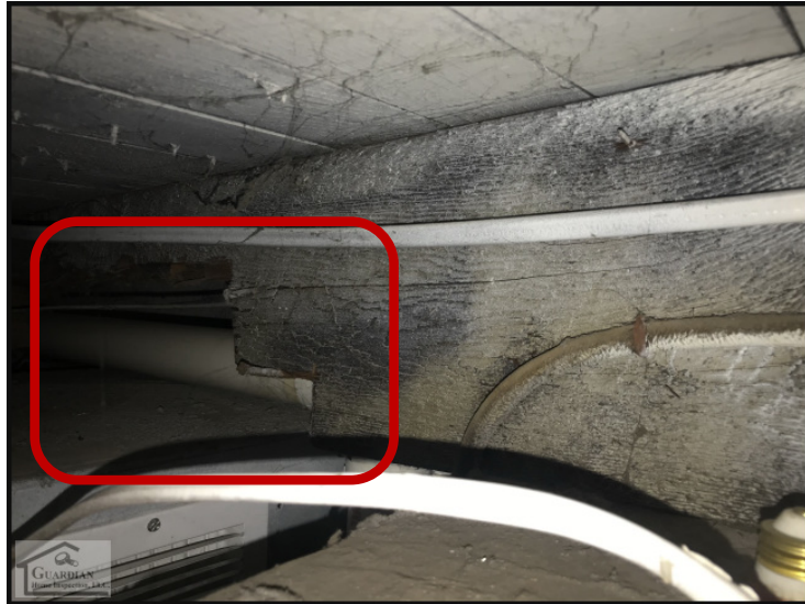
Figure 33 A wooden floor joist, along the basement ceiling (above the furnace) has been excessively notched.
