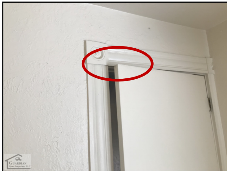
Figure 18 The 2 nd floor west facing bedroom door does not open/close smoothly and should be trimmed or adjusted as necessary.
