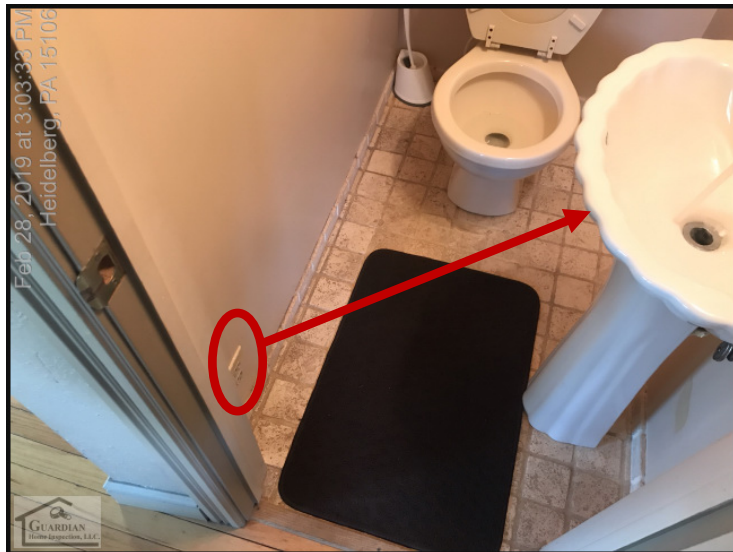
Figure 44 The home lacks adequate Ground Fault Circuit Interrupter (GFCI) outlet protection in the powder room.
