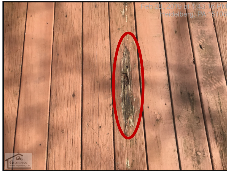
Figure 3 Several of the wood planks, on the exterior decking, exhibit signs of moisture related rot.
