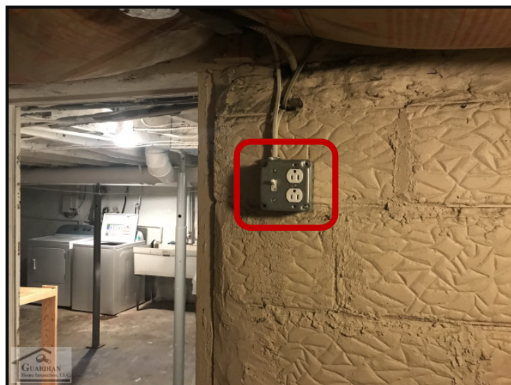
Figure 30 The home lacks adequate Ground Fault Circuit Interrupter (GFCI) outlet protection in the unfinished basement.
