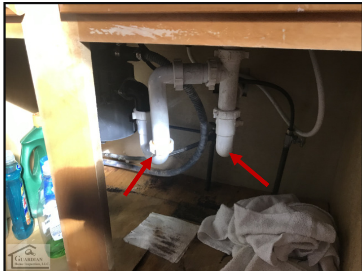
Figure 50 The drain lines, under the kitchen sink, are double trapped.
