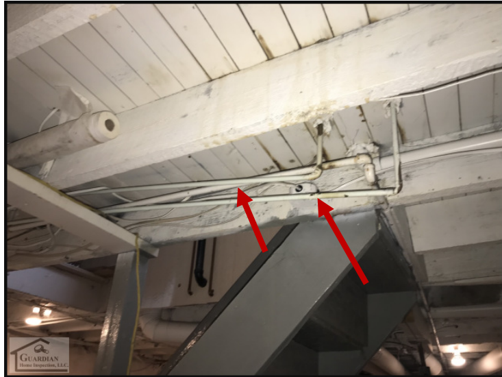
Figure 41 The water distribution piping, along the basement ceiling, is poorly supported in some areas.
