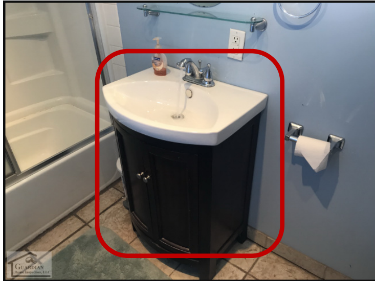
Figure 19 The second-floor hallway bathroom sink and cabinet are not well secured to the adjacent wall.
