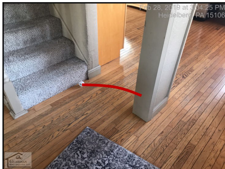
Figure 46 Areas of the flooring, along the first floor (at the base of the 1st floor stairway), are unlevel and sloping.
