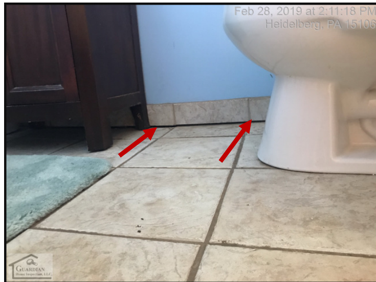
Figure 21 The wall tile, in the 2 nd floor bathroom, has separated from the floor tile against the north facing wall
