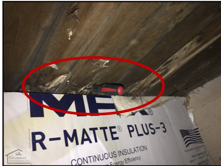
Figure 29 An area of the sub-flooring, along the basement ceiling (below the north facing entry door), exhibits evidence of moisture related rot.
