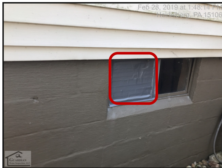
Figure 8 A window pane, along the north facing basement wall, is damaged and requires replacement.
