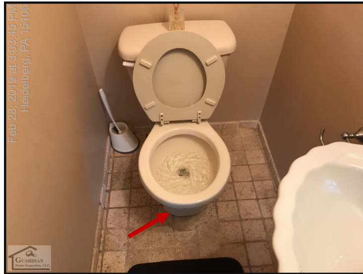
Figure 45 The toilet, in the powder room, is loose from the floor.
