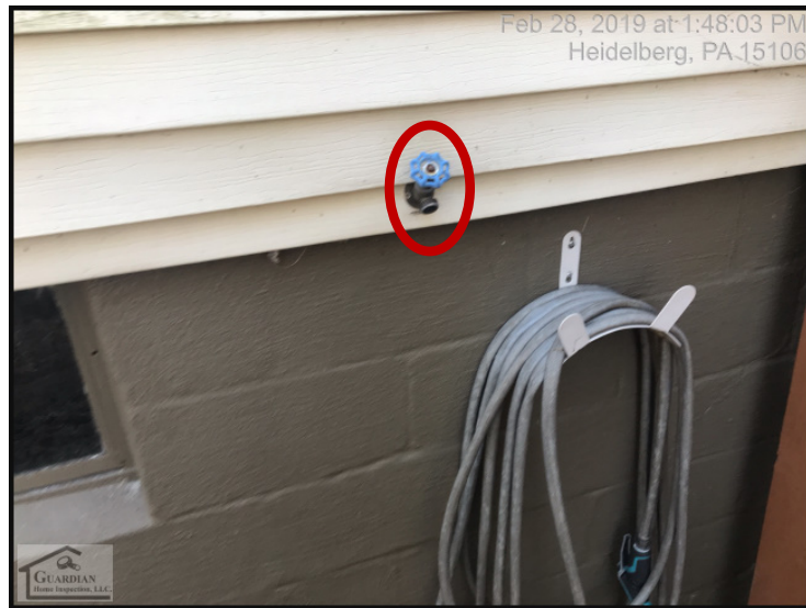
Figure 7 The exterior hose faucet lacks and anti-siphon device.
