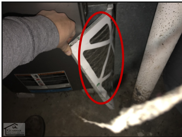
Figure 36 The dirty air filter, serving the furnace and air conditioner, should be replaced.
