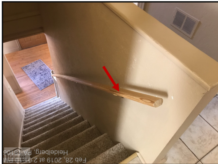
Figure 16 The handrail, on the first-floor stairway, is loose/unsecured; repair is recommended.
