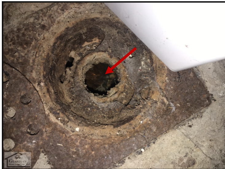
Figure 40 Because back-up or blockage in the drain lines sometimes takes extended periods of time to develop it is highly recommended that the overall inspection of the plumbing system includes a sewer cam inspection of the underground sewer lateral.
