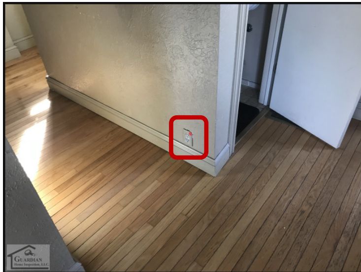
Figure 42 Several of the three-prong electrical outlets, in the home, are ungrounded and have been labeled with red stickers.
