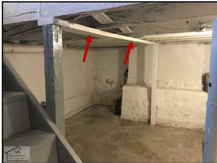
Figure 26 The floor framing, along the basement ceiling, has been reinforced in several locations with central support framing.
