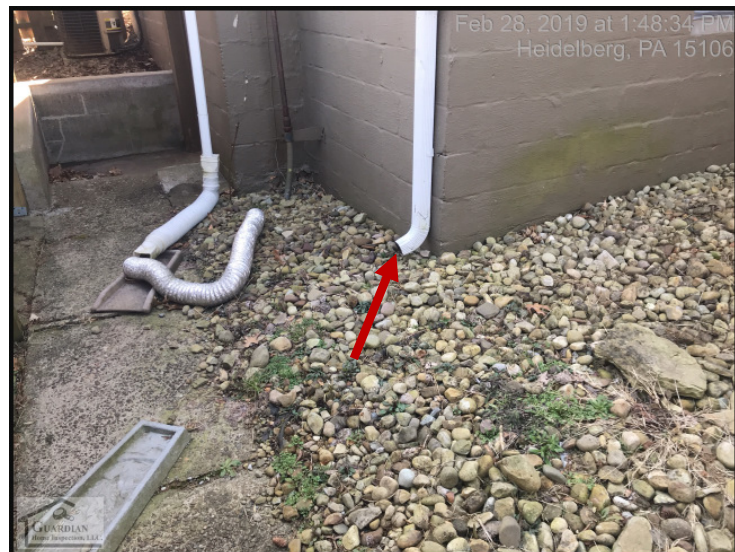
Figure 6 The gutter downspout, at the northeast exterior corner of the home, should discharge further away from the foundation.
