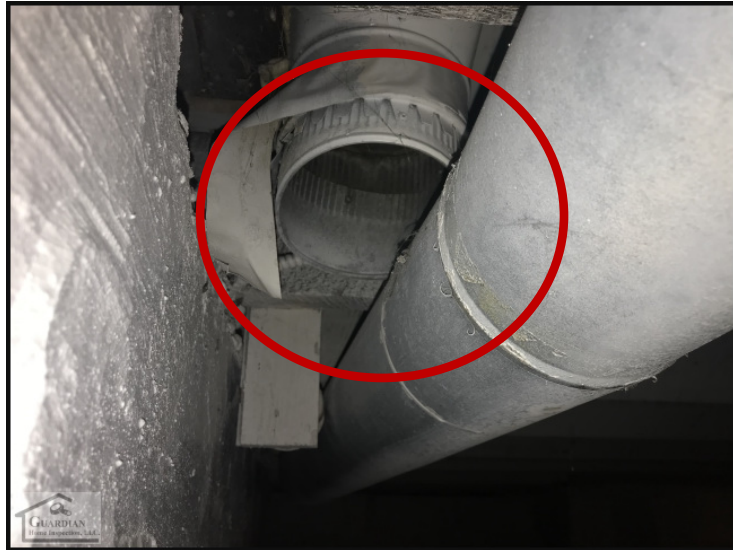
Figure 37 The disconnected supply ductwork, along the basement ceiling, should be reconnected to prevent air leakage and to improve overall balancing of the system.
