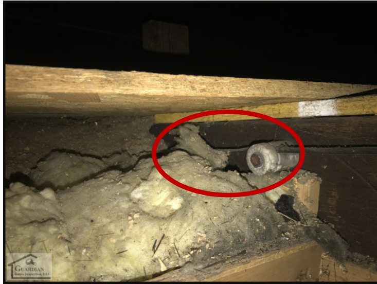
Figure 23 Active knob & tube wiring was observed in the attic covered with insulation.
