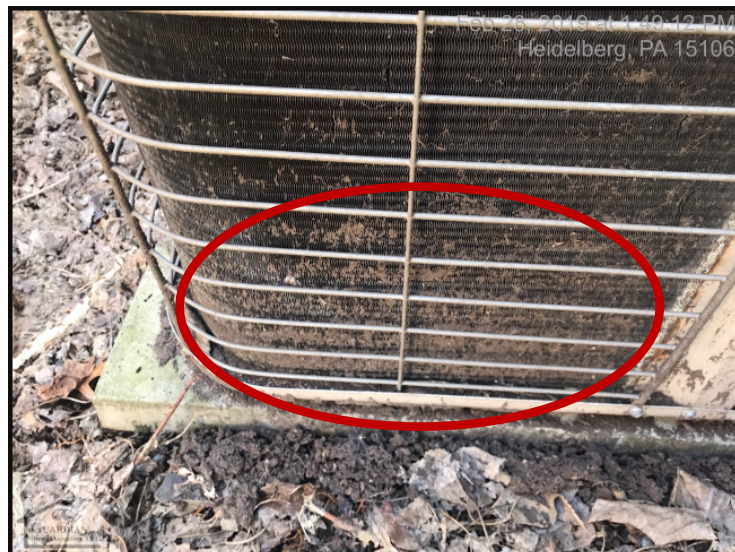
Figure 10 The condensing coil fins, on the exterior AC unit, are significantly dirty.
