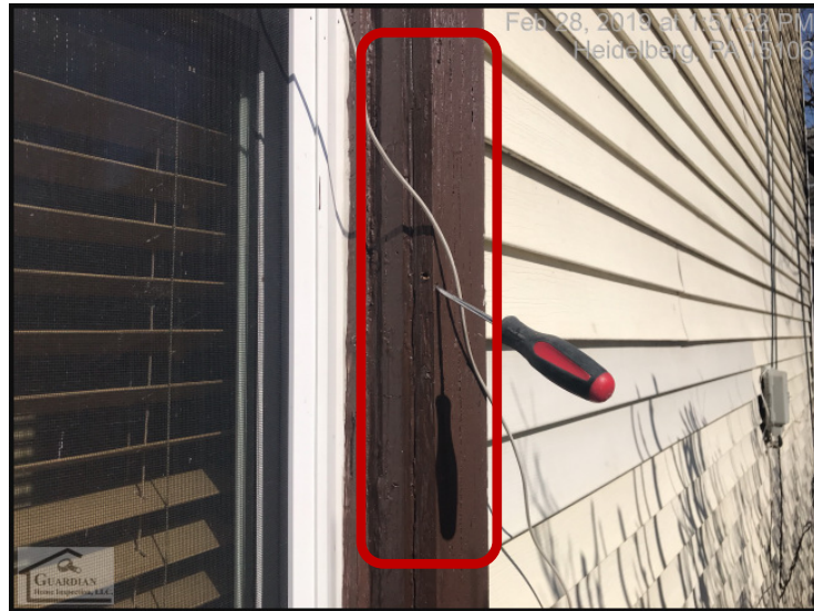
Figure 13 Most of the exterior wood window trim, framing and sills are significantly moisture rotted and should be replaced, painted and caulked.
