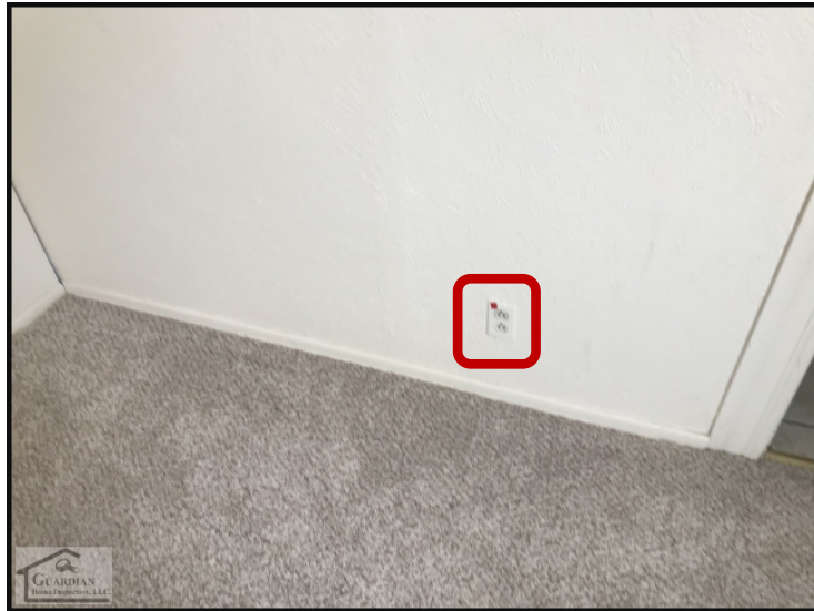
Figure 17 Several of the three-prong electrical outlets, in the home, are ungrounded and have been labeled with red stickers.
