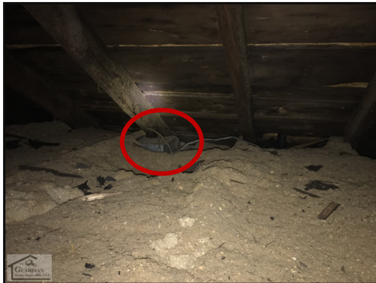
Figure 24 The bathroom exhaust fan is exhausting into the attic.
