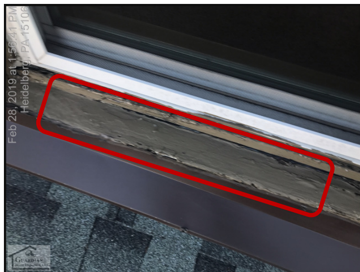
Figure 14 Most of the exterior wood window trim, framing and sills are significantly moisture rotted and should be replaced, painted and caulked.
