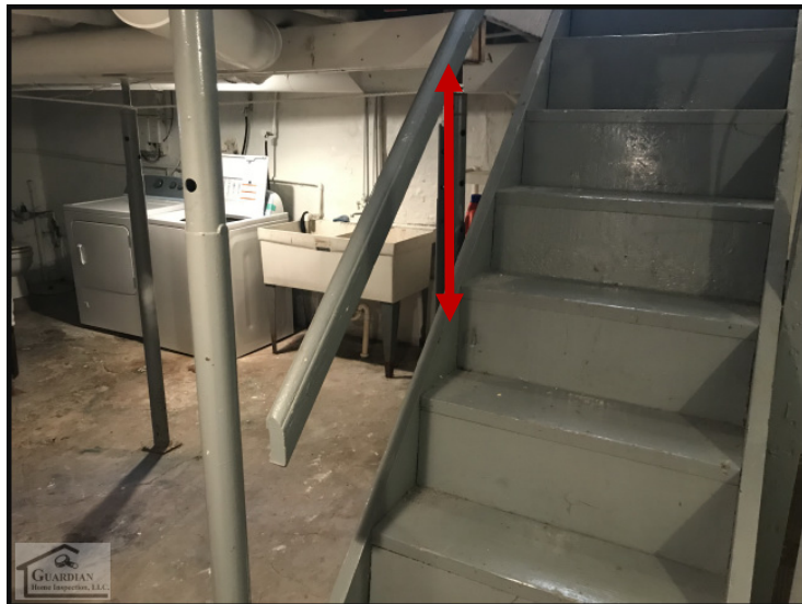
Figure 32 As there is a danger of falling, a step railing should be provided along at least one side of the basement stairway.
