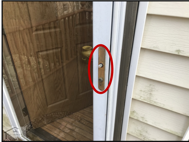
Figure 52 The door handle hardware, on the north facing storm door, is damage/missing.
