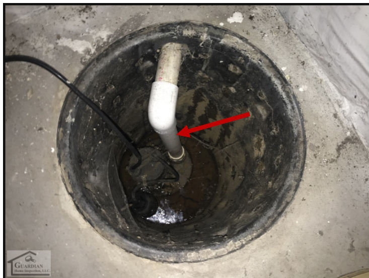
Figure 38 The sump pump has no visible check valves installed along its discharge piping.
