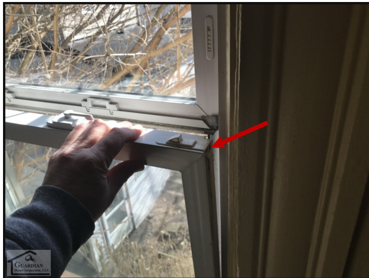
Figure 20 The tilt latches, on the 2 nd floor southeast facing bedroom window, are broken.
