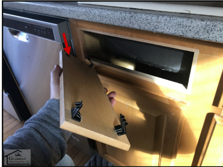
Figure 51 The retaining clip, on the cabinet face plate along the front of the kitchen sink, is damaged and in need of replacement.
