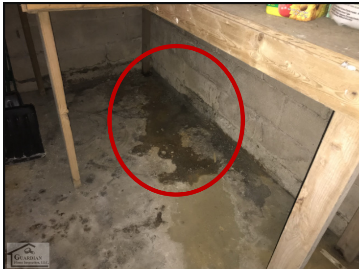
Figure 28 The interior north facing basement foundation wall exhibited evidence of moisture infiltration and staining/efflorescence.
