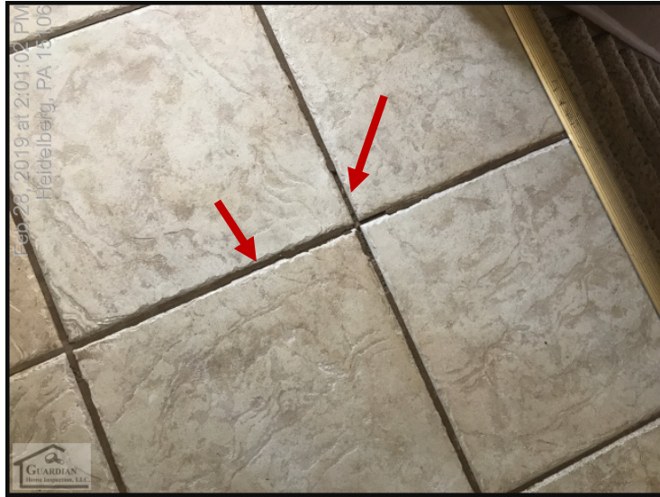
Figure 15 Some areas of missing grout were observed along the floor tiles in the 2 nd floor hallway.
