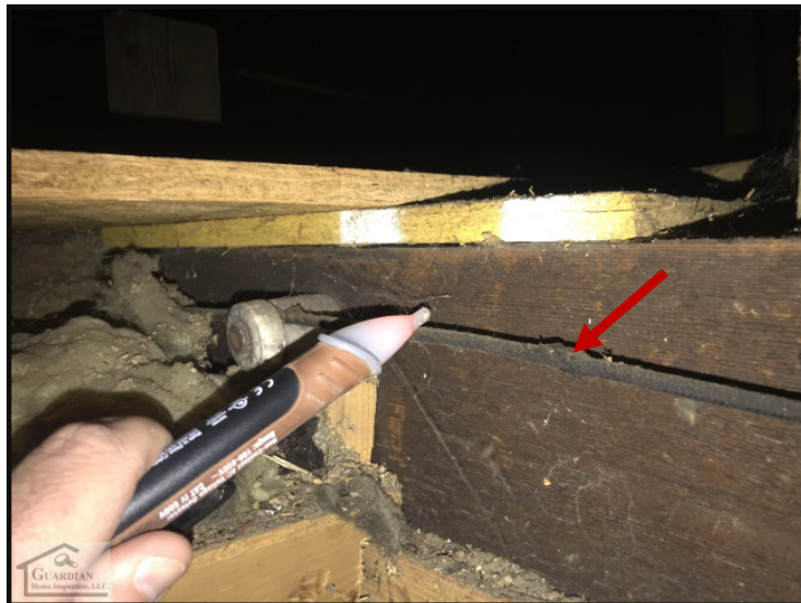
Figure 22 Active knob & tube wiring was observed within the attic space.
