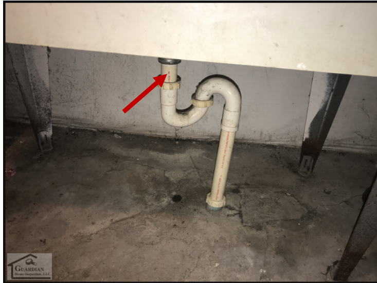
Figure 39 The drain piping, under the utility sink in the basement, was actively leaking at the time of inspection.
