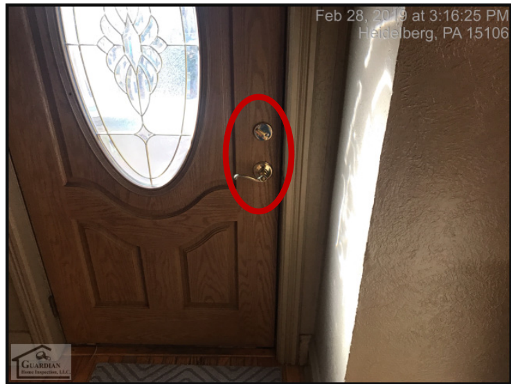
Figure 47 The locking hardware, on the west facing entry door, is need of repair (the dead bolt, latch and striker plate are misaligned preventing the door from locking).
