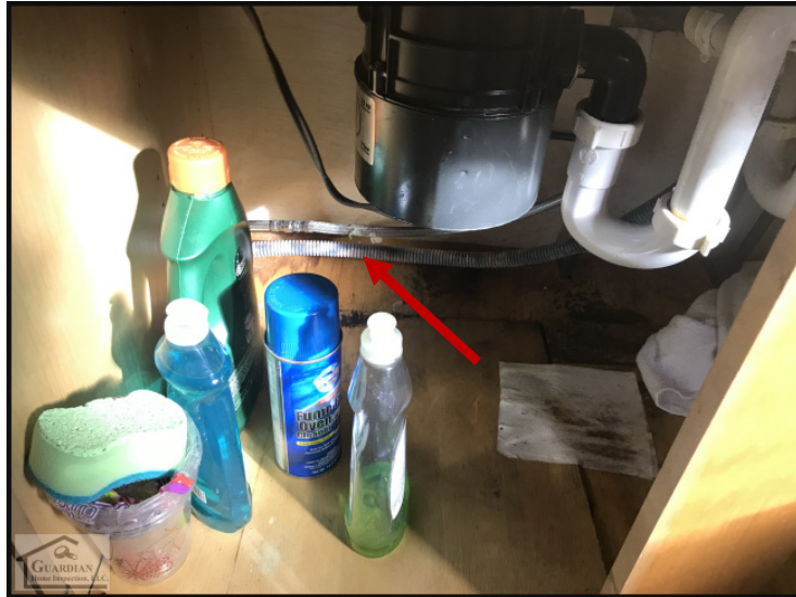
Figure 49 The dishwasher's discharge line has no visible high-loop installed.
