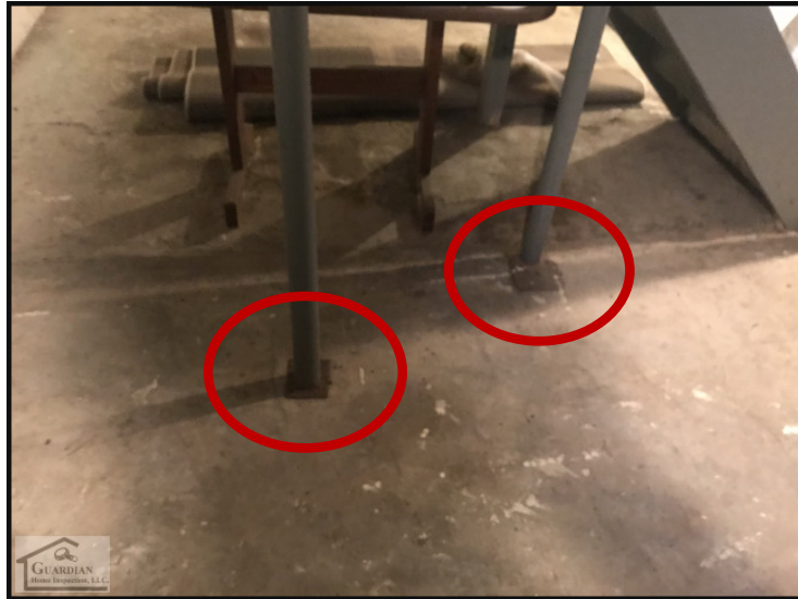
Figure 27 The reinforcing vertical support posts do not appear to have underlying concrete footers installed.
