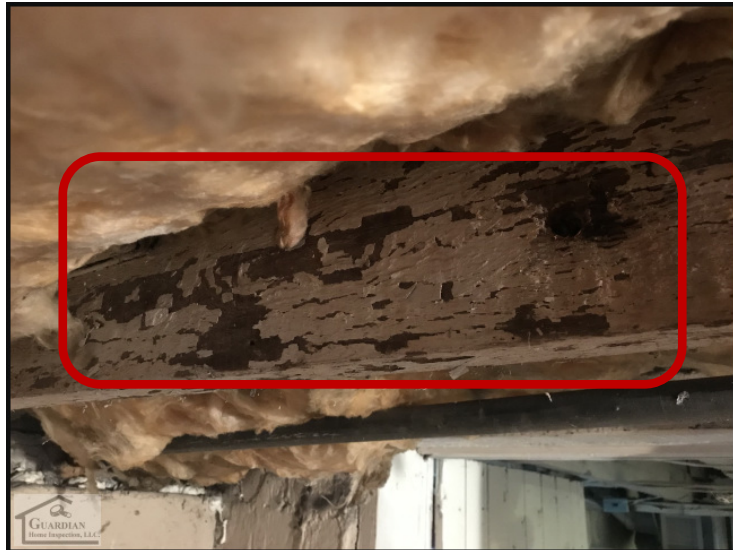
Figure 31 Based on the age of this home, there is a possibility the peeling paint, on the floor joists along the basement ceiling, may contain some lead based paint.
