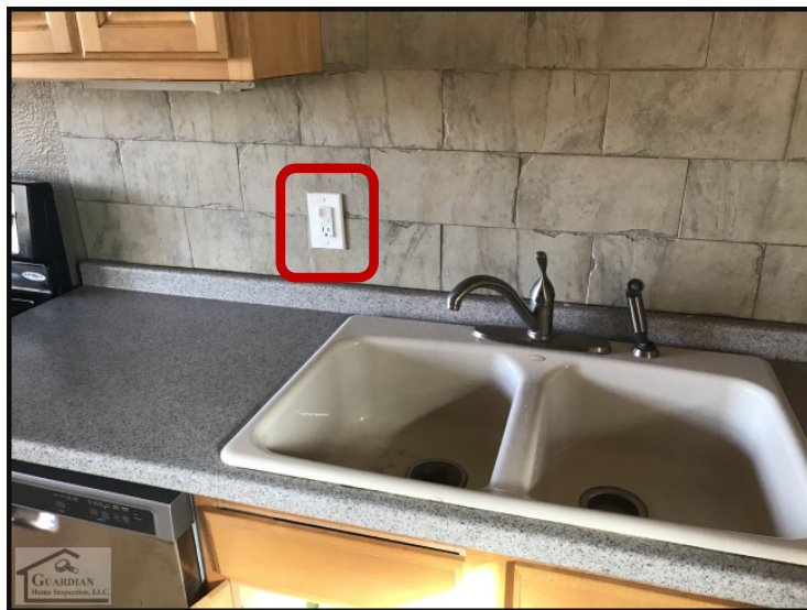
Figure 48 The ground fault circuit interrupter (GFCI) outlet, along the left hand side of the kitchen sink, was inoperative (not tripping/resetting) at the time of inspection.
