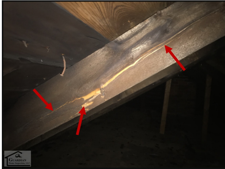
Figure 25 A wooden roof rafter, along the south facing slope of the attic, has cracked the extent of its depth.
