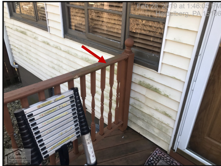
Figure 5 The wood guard railing, on the deck, is significantly loose (next to entry door) and should be adequately resecured.
