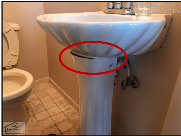
Figure 43 The pedestal sink, in the powder room, is not well seated into the underlying pedestal.
