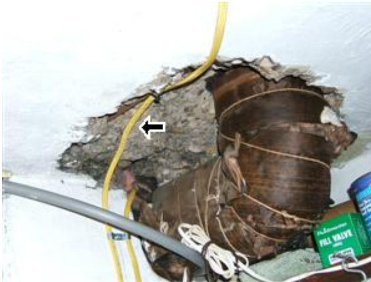
4.5 WALLS / CEILINGS Picture 1
