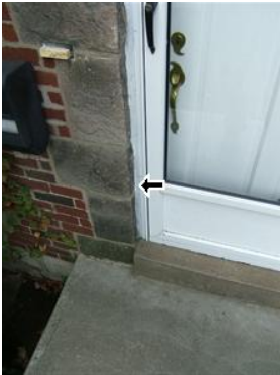
2.3 ENTRY DOORS Picture 1
