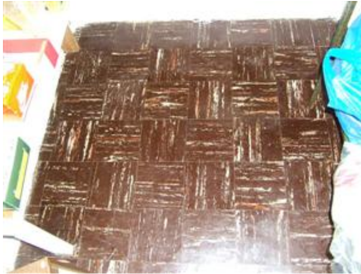
9.4 BASEMENT FLOOR (SLAB) Picture 1
