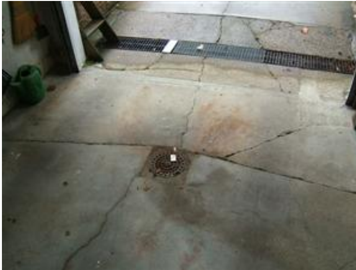
4.2 FLOOR SLAB Picture 1
