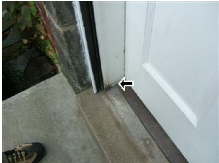
2.3 ENTRY DOORS Picture 2
