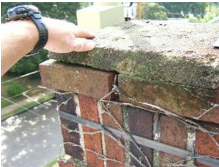
1.1 CHIMNEYS / VENTS Picture 1
